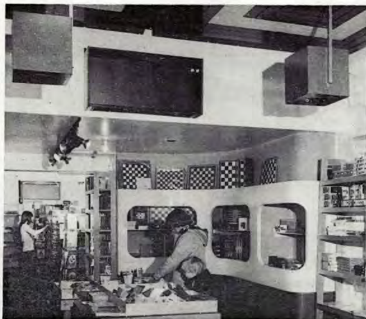
Up above the customers, the cleverly planned air-conditioning equipment.
